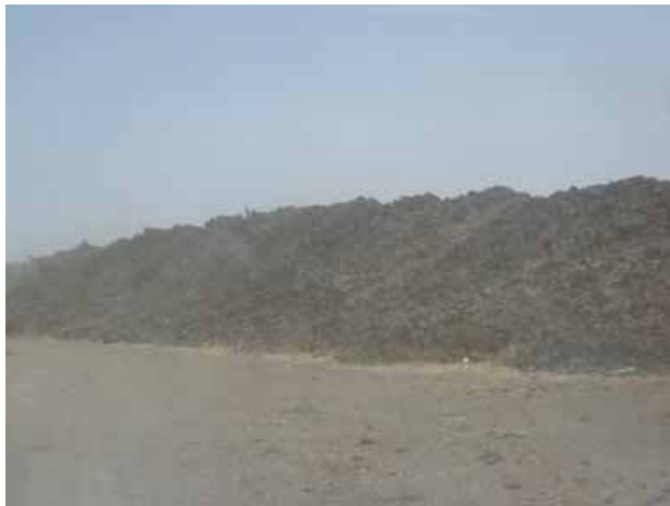
FIGURE 29. Sedimentation challenges in canals of 80 km Meana to Rahad conveyance. Note the canal is behind the pile of dredged sediment ( photo credit: Seleshi B. Awulachew ).
