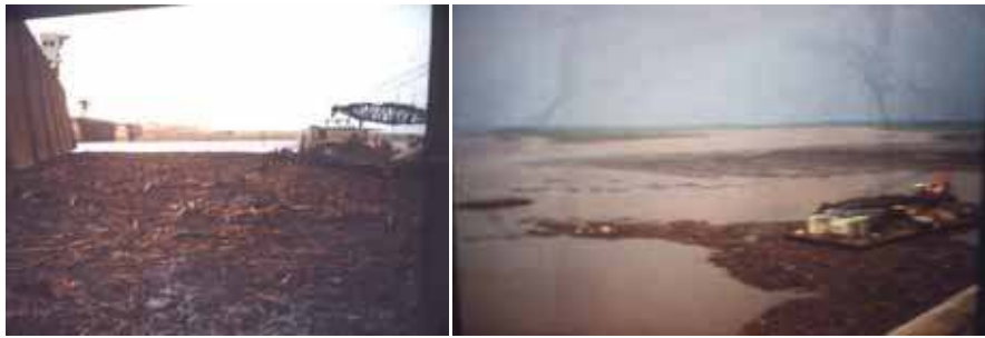
Figure 27(a). Delta formation upstream, Roseries Dam (Photo: Ahmed 2005); (b) Debris in the reservoir upstream, Roseries Dam (Photo: Ahmed 2005).
