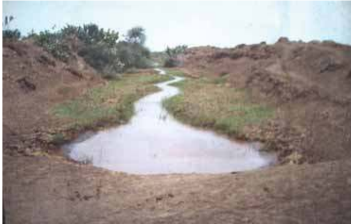
FIGURE 28. Sedimentation problem in the Gezira scheme canalization system ( photo credit: Abdella A. Ahmed ).
