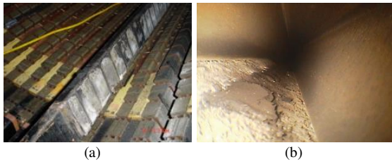
Figure 6. (a) The fault scene of the spark discharge after the stator bar near the neutral point of the winding is removed, (b) Borescope images of the side of a stator bar surface damaged by vibration sparking [23].
