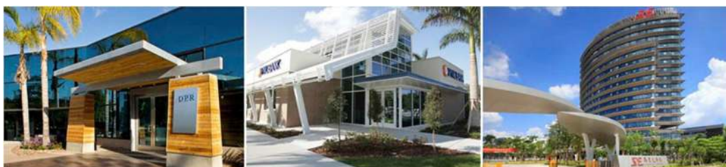
Fig. 12. Three NZEB cases: U.S. bldg. 1 (left, NBI 2018), U.S. bldg. 2 (middle, NBI 2018), Xingye building (right).
