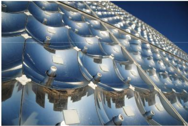
10 11 12 13 14 15 16 17 18 19 20 21 22 23 24 25 26 27 Figure 9: Concentrated PV (CPV) cells [120]
