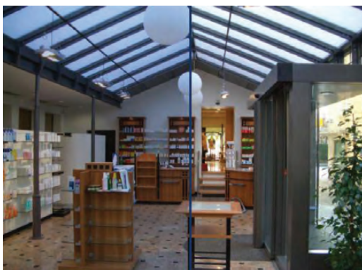
Figure 4. Translucent aerogel roof in a pharmacy of Switzerland [21].
