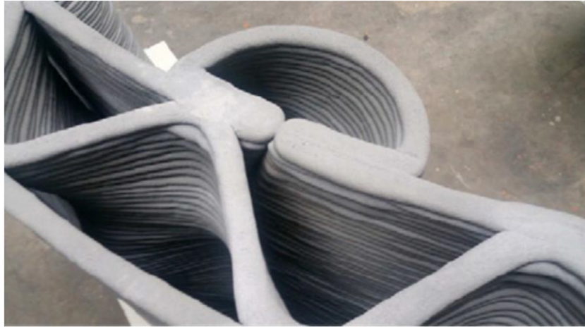
Fig. 14 – Layered appearance defect in concrete structure obtained via AM route [281].
