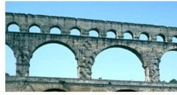
(b) Ancient arch structures
