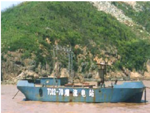
Fig. 3. 70 kW tidal current energy plant.
