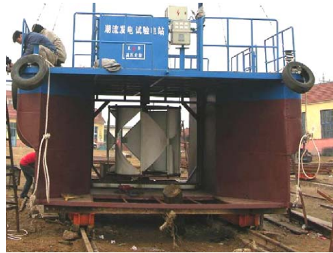
Fig. 5. 5 kW tidal turbine by OUC.
