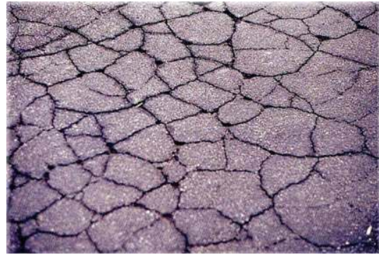
FIGURE 11: Fatigue cracking.
