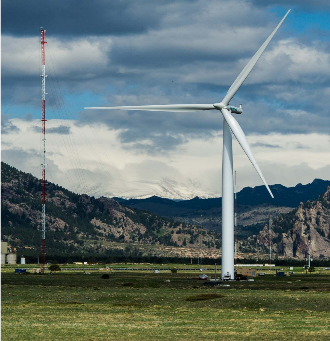
Figure 1.3: Typical Horizontal Axis Wind Turbine ((Golden, Colorado); courtesy of DOE/NREL, credit – Dennis Schroeder, PIK # 25907) www.nrel.gov .
