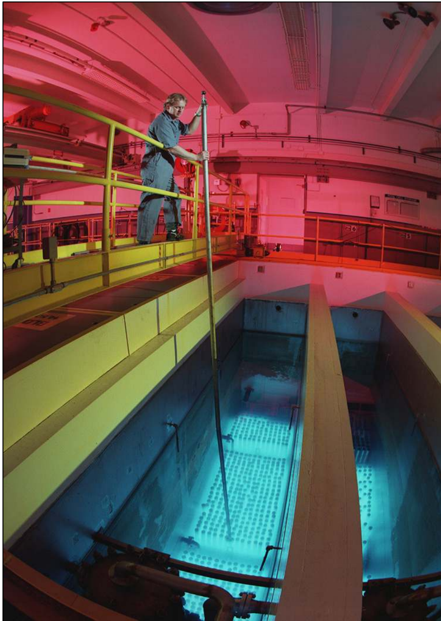
Cesium and Strontium Capsules. Water-filled pools inside the Waste Encapsulation and Storage Facility, adjoining B Plant, contain 1936 stainless-steel capsules holding intensely radioactive cesium and strontium.
