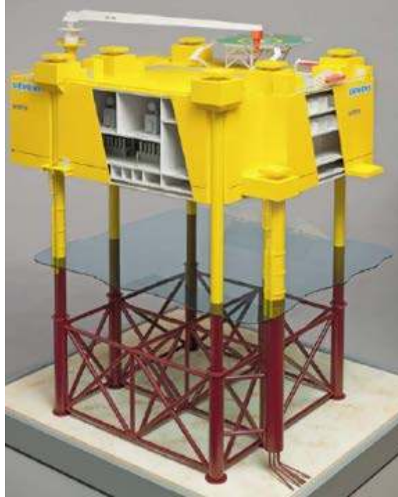
Figure C-23. Siemens Helwin HVDC platform. Image from Siemens Energy
