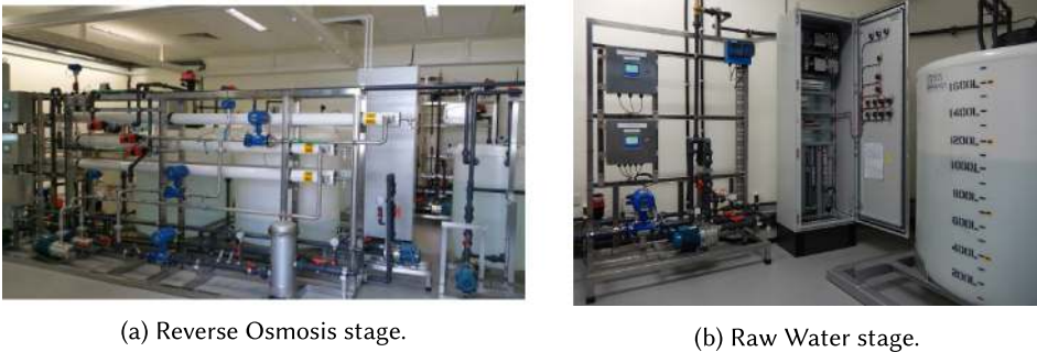
Fig. 11. Illustrations of the SWaT testbed.
