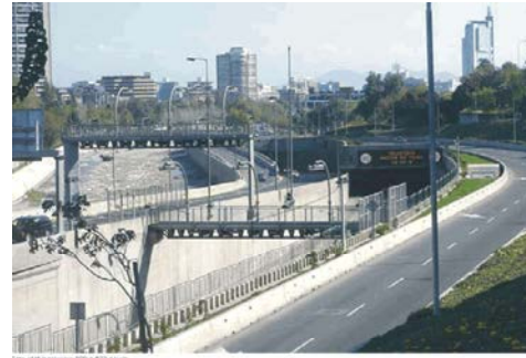
Fig. 2: Electronic toll collection at Costanera Norte Freeway [18]
