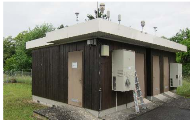
Fig. 3. Governmental monitoring station located in a suburban area in Switzerland.
