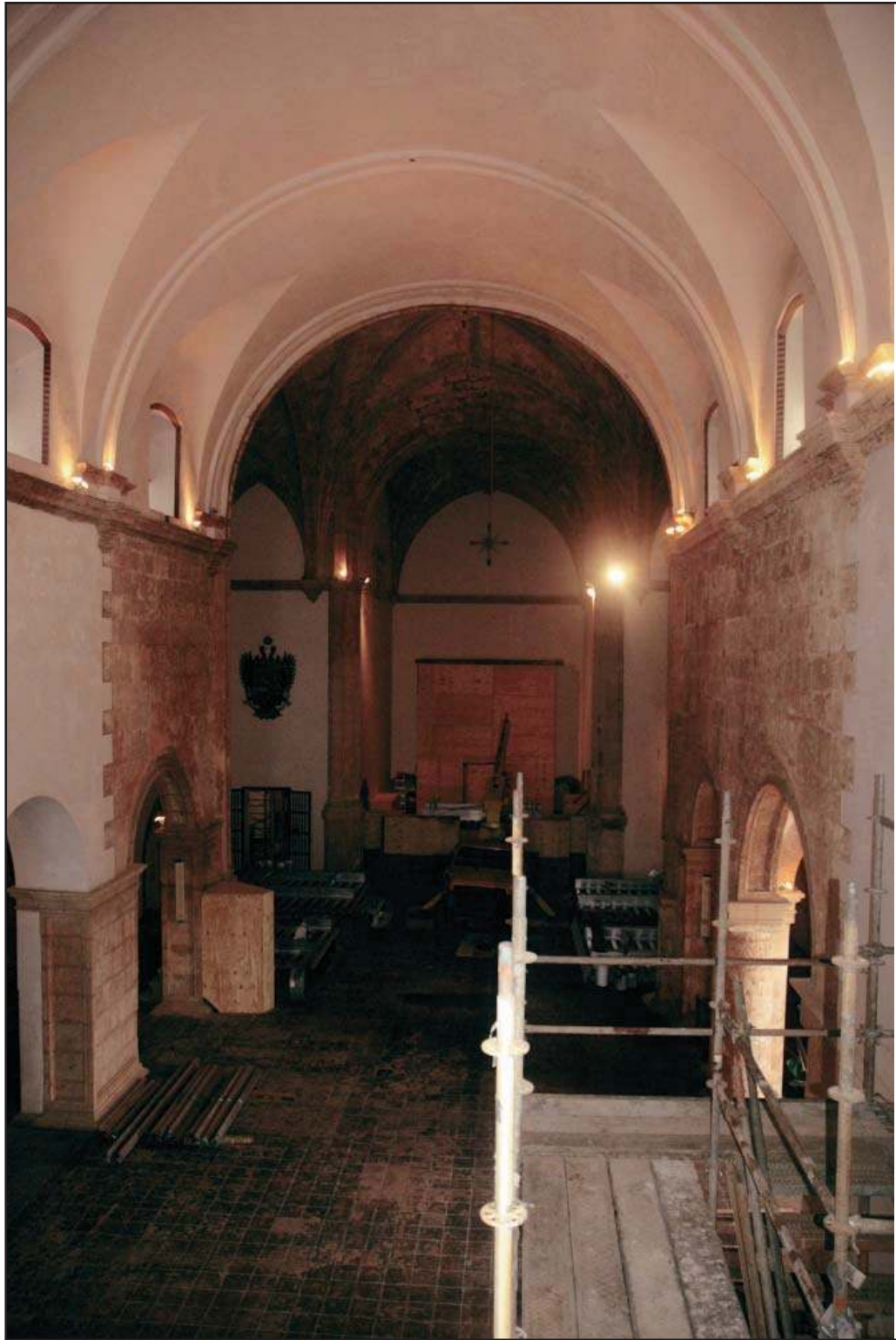
Figure 5: View of nave barrel vault from the choir loft. Rosario Chapel to the rear right. (Source: C. Silva, 2006)
