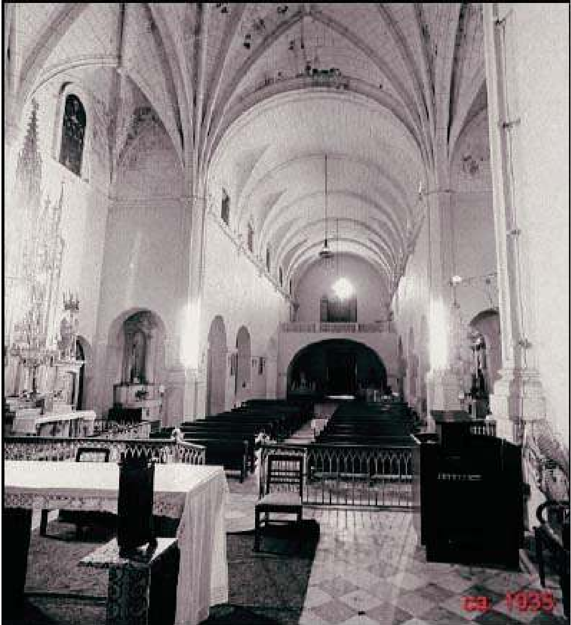
Figure 9: Circa 1935 photograph taken from the sanctuary looking toward the nave. (Source: HABS, PR, 7-SAJU,1-20)
