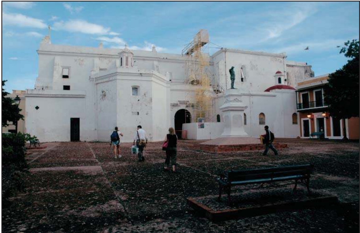
Figure 12: South elevation of Iglesia San José, Rosario Chapel located west (left) of the scaffolding. (Source: C. Silva, 2005)
