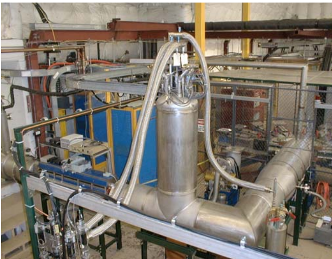
Fig.6. A view of the magnet test system. From left to right: 180 deg. return conductor, magnet with field measuring instrumentation, liquid helium feed & instrumentation tower, and 90 deg. bent conductor followed by current leads and assembly of rectifiers.
