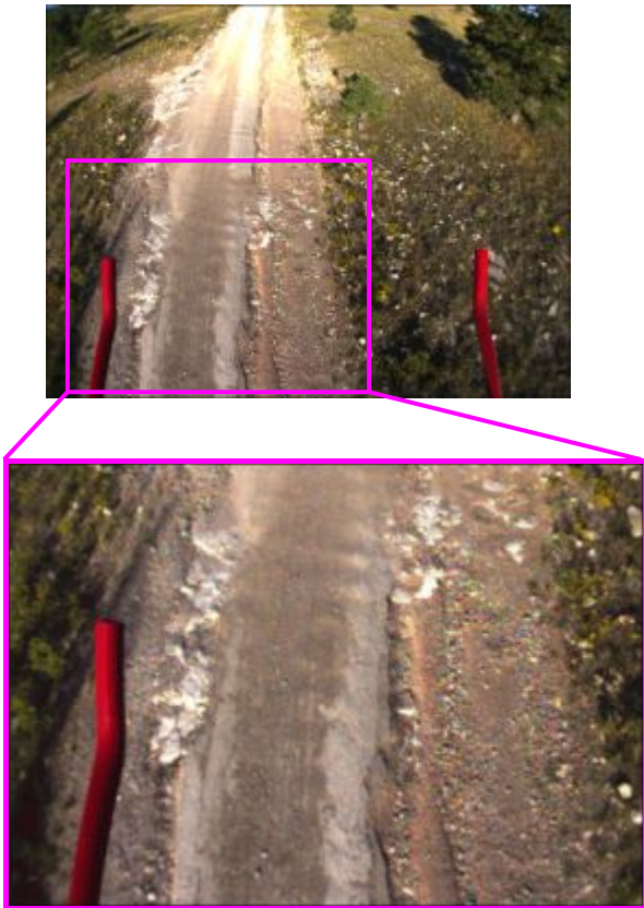
Figure 4. An image of a road segment with serious distresses collected from the UAV platform.
