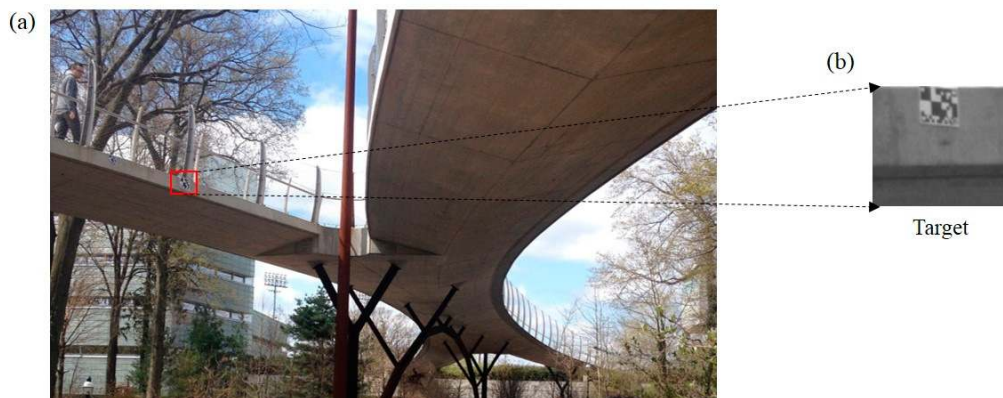
Figure 14. Field test: (a) Streicker Bridge; (b) Artificial target.
