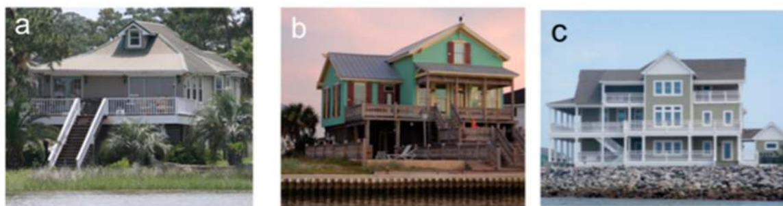
Figure 1. Photographs of waterfront homes with shorelines representing natural (a), vertical wall (b), and rip-rap revetment (c) shorelines. Photo Credits: S. Scyphers (a,b) and R. Gittman (c).
