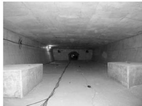
(c) Interior of the box girder.
