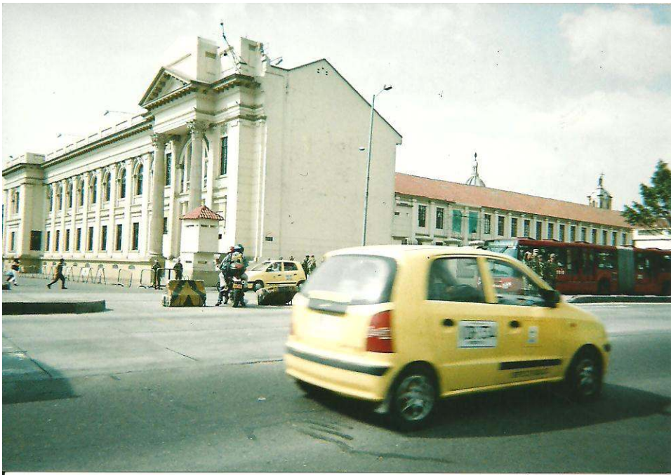
Photograph 5.5: La ‘L’ – Military Barracks
