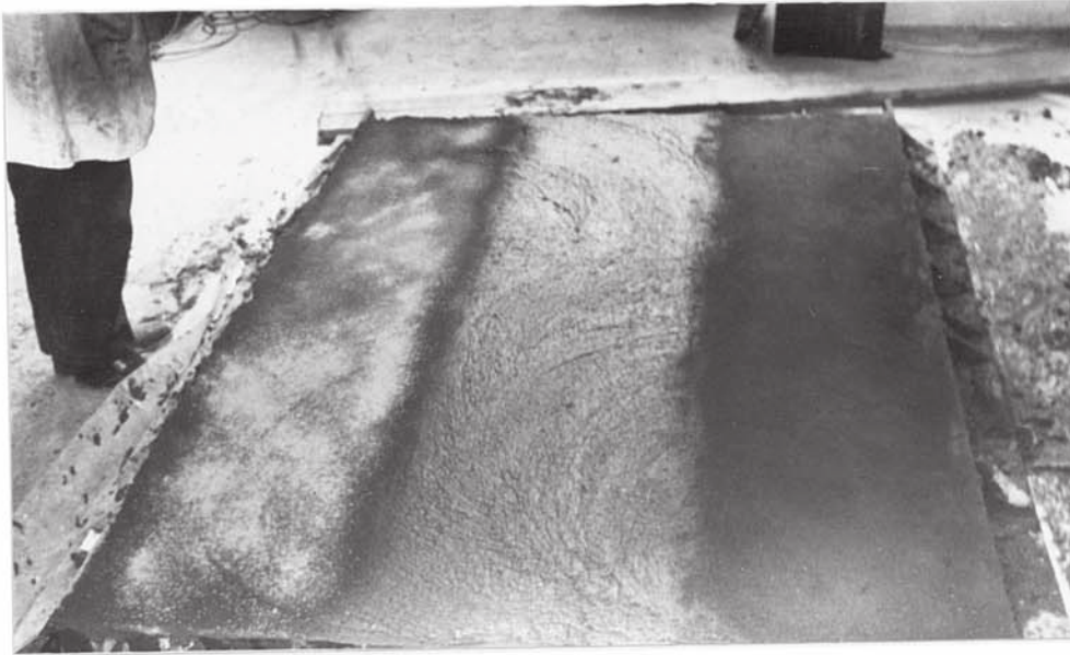
Plate 6.7 Application of Dry Shake Surface Treatment
