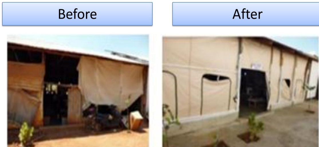
Figure 3 (b) Exterior Appearance of the Enterprise Before and After 5S-KAIZEN
