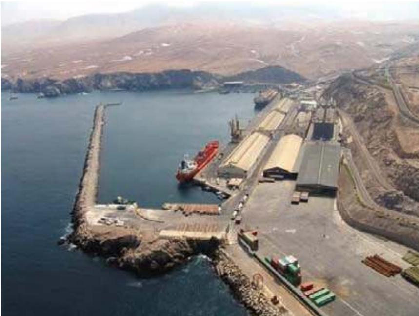
Figure 5.2: Matarani Port Terminal (Peru)
