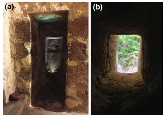
Fig. 5 In this picture, a small cabin in the wall contains a hole pointing downwards. (a) The hole acts as a pinhole projecting a green patch on the ceiling. (b) View outside the hole. This hole was used as a toilet by the guard of this jail of the XVI century in Pedraza, Spain
