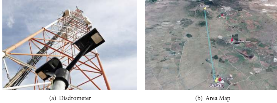
FIGURE 1: The installed OTT Parsivel Disdrometer Weather Sensor near Ortal's MCN base-station tower (a), and the test area map showing the ML's 12.08 km path, as well as the three available RGs: RG-Ortal , RG-Merom-Golan and RG-El-Rom (b). (Image (a) was taken by Y. Dagan. Image (b) was created via Google Earth).
