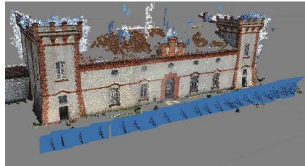
Figure 9. Camera positions for the survey of the front façade.
