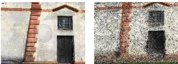
Figure 20. The images above show the difference between the point cloud of model M3 (on the left) and the one obtained from the unique model (on the right). The comparison shows the higher definition of the first one.
