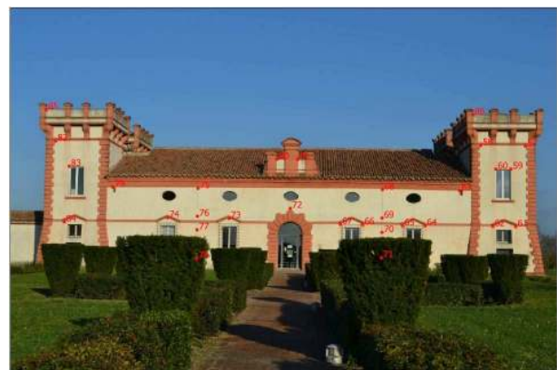
Figure 4. Location of control points on the main façade of the Castle
