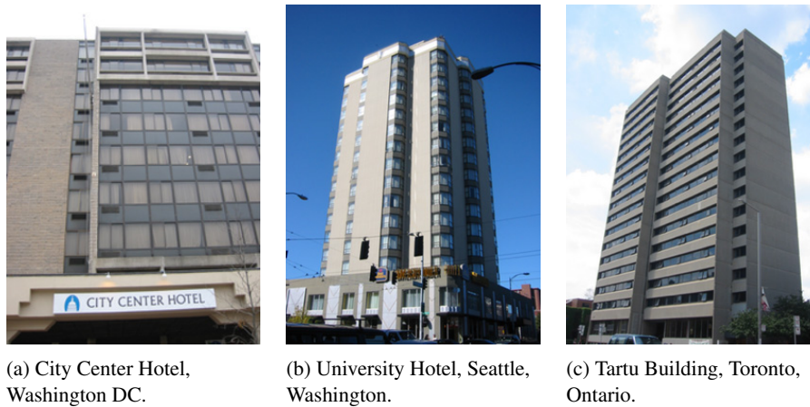
Fig. 9. The tall multi-floor buildings where the data was collected.
