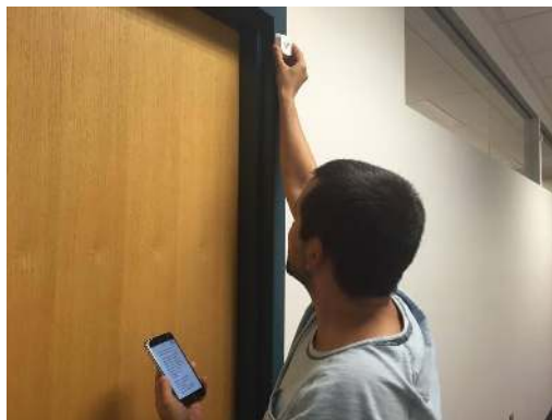
Figure 1: Beacon installation is performed by expert personnel.
