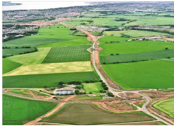
Fig. 1. A92 PFI road project under construction (Courtesy: MorganEST Rugby Office Archive)
