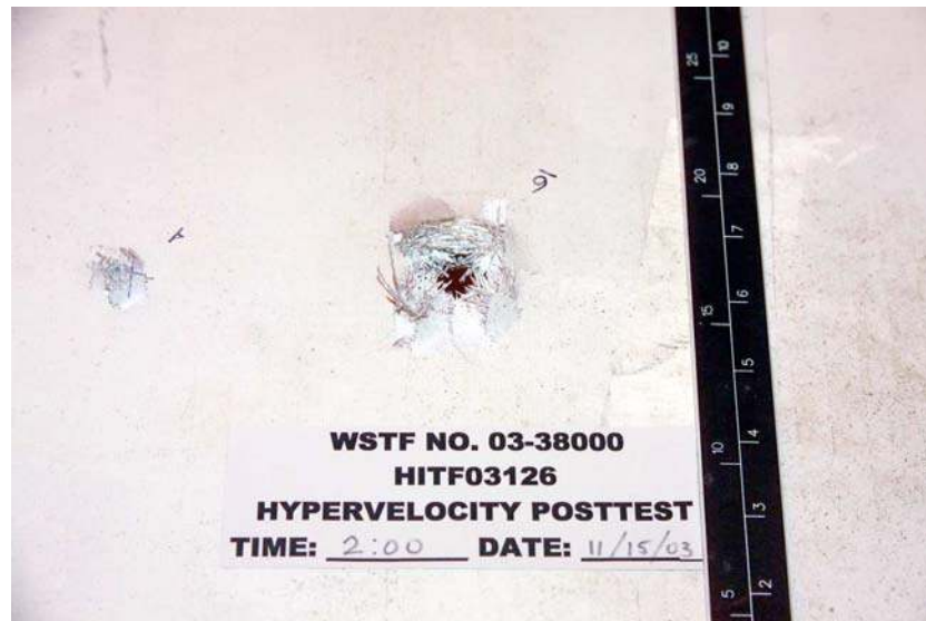
Fig. 5 Fiberglass panel showing damage from two hypervelocity impacts.
