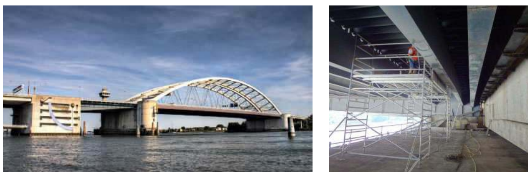
Figure 9. Van-Brienoord bridge in Rotterdam (left); installation of the sensors (right).
