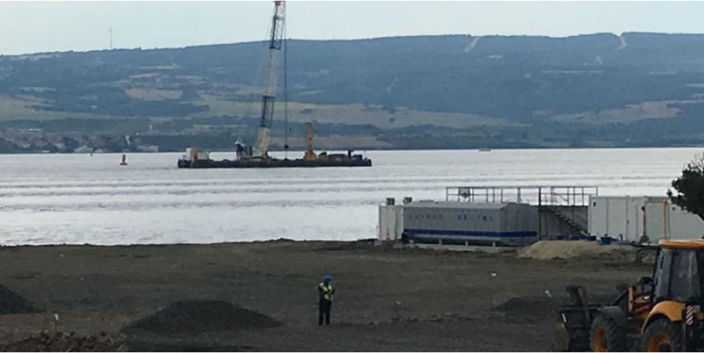
Photo 1. Pile driving platform at operation for suspension bridge construction (original)
