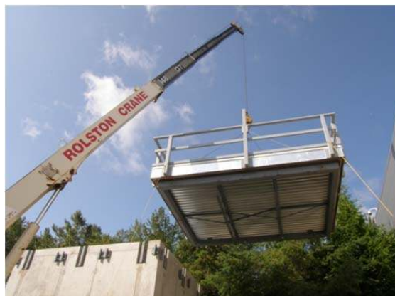
Figure 32 Hoisting of test panel onto sound transmission suite
