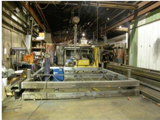
Figure 30 Construction of test roofs A and B
