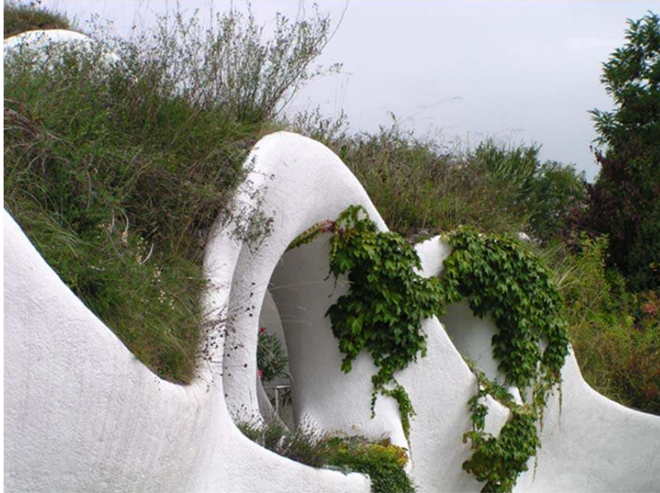
Illustration 6 Multi-family residential, Lattenstrasse, Switzerland Architect Peter Vetch
