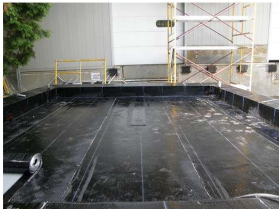
Figure 31 Installation of roofing materials on test roof A
