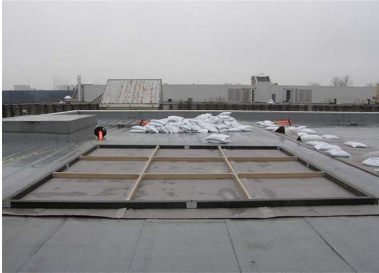
Figure 11 In-situ plots under construction – drainage layer and frame
