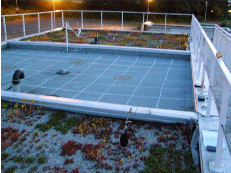
Figure 24 Field test facility, non-vegetated roof and two vegetated roofs
