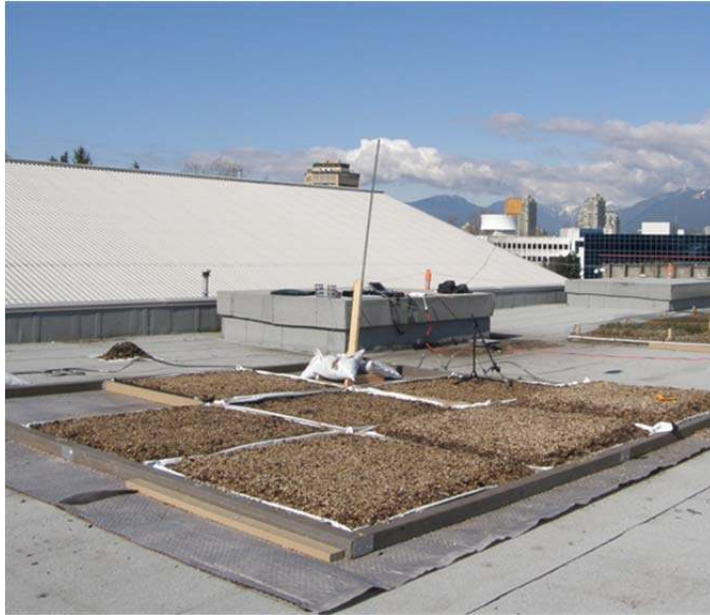
Figure 13 In-situ plots-substrates measurements, September 2010
