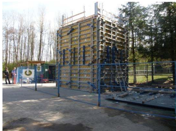
Figure 29 Construction of indoor-to-outdoor sound transmission suite
