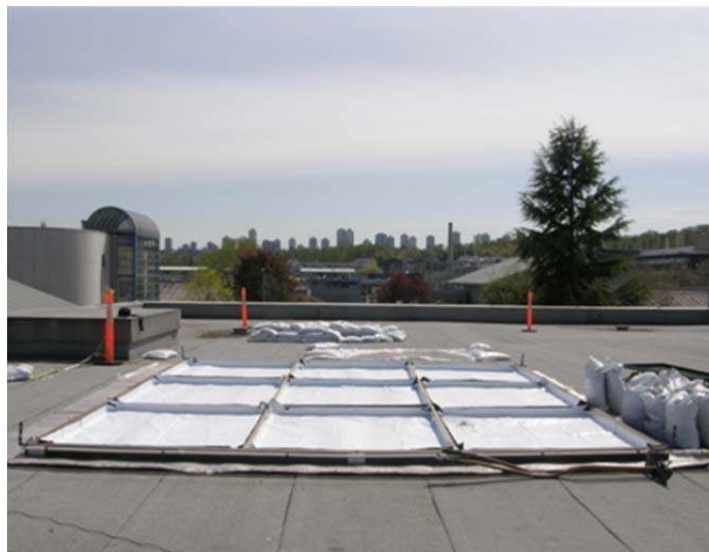
Figure 12 In-situ plots under construction – filter cloth / root barrier
