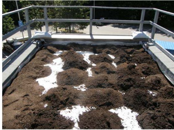
Figure 33 Installation of first 50 mm depth of substrate over filter fabric
