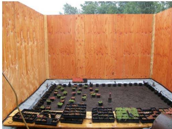
Figure 34 Planting of sedums (P1) on test roof A
