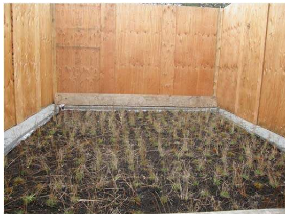
Figure 35 Completion of planting of coastal community on test roof B
