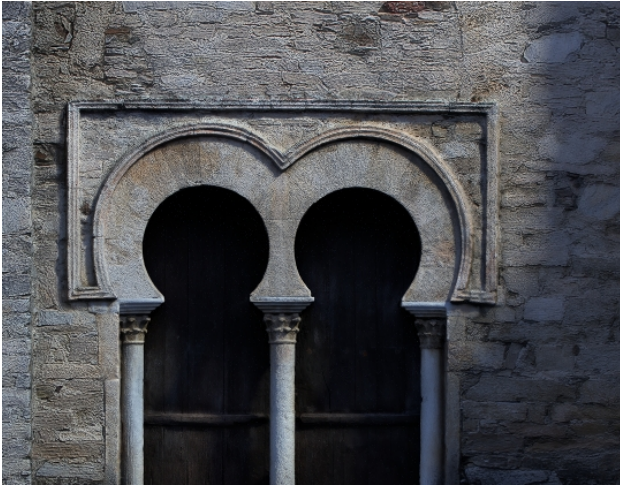
Figure 16: Door of Santiago de Peñalba, Leon, Spain. Detail of the orthoimage(down) with slightly different slanted illumination to highlight relief details.
