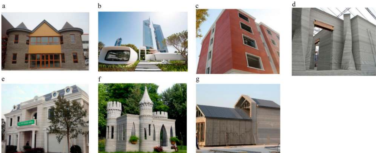
Figure 3. Noteworthy examples of projects using AMoC: (a) Two-storey house in China by HuaShang Tengda, (b) Office building in Dubai by Winsun, (c) five-storey building in Suzhou, China, by Winsun, (d) Hotel suite interior in the Philippines, by Total Kustom, (e) Villa in Suzhou by Winsun, (f) Castle in Minnesota, USA, by Total Kustom, and (g) series of 10 houses in Suzhou, by Winsun.
