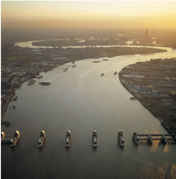
Fig. 1 The Thames barrier ( bottom of photo). Source: Environment Agency
