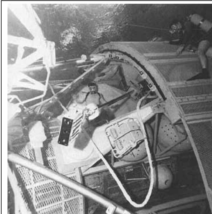
Figure B.5-2. Activities on 5 January 1972 during a simulation of film retrieval from the Apollo Telescope Mount (Skylab) in the Marshall Space Flight Center Neutral Buoyancy Simulator.
