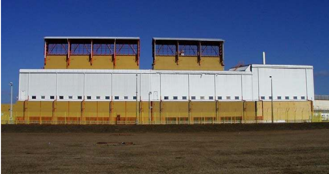
Figure A-6. Paks MVDS in 2000 showing natural convection cooling exhaust outlets (Ordogh et al. 2004).
