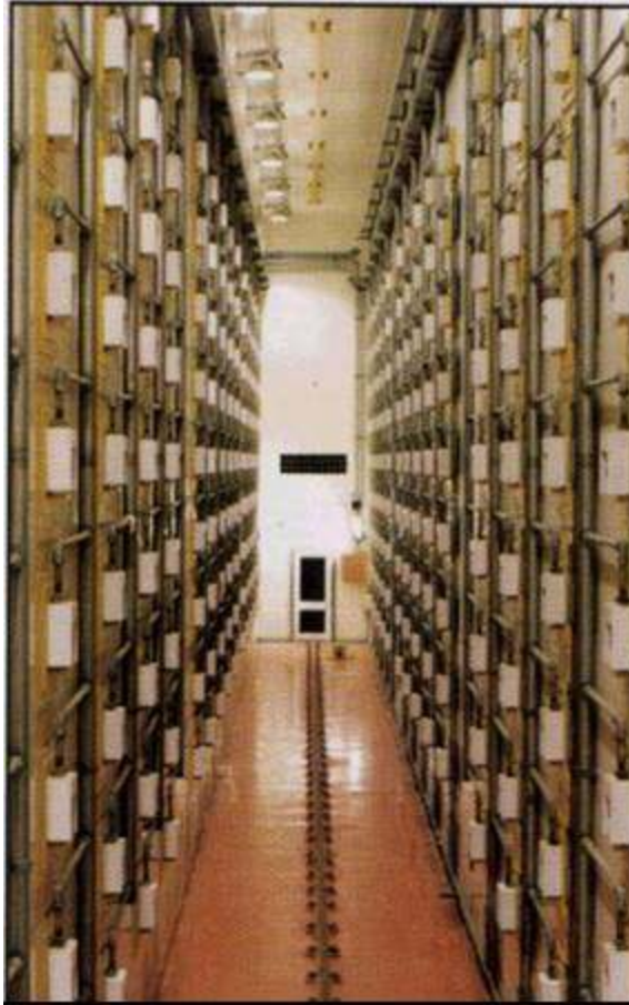
Figure B-1. Remotely operated store for Pure \text{PuO}_2 in welded stainless steel canisters at BNFL Sellafield.
