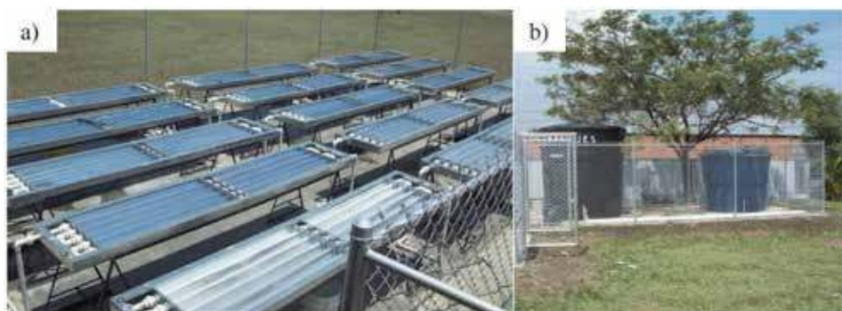
Figure 18. Full-scale solar photocatalytic plant for dye-polluted wastewater treatment: (a) CPC photoreactors and (b) recirculation-feed and treated water storage tanks.
