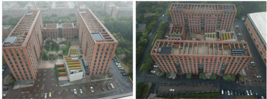
Figure 13. Drone images of the building image set.
