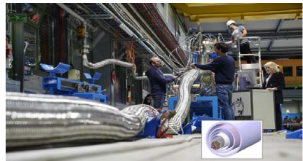
Fig. 3 Superconducting cable assembly 14) .
