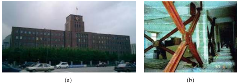
Figure 7: Shenyang Government Office Building retrofitted by friction dampers.
