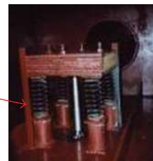
Figure 20: TMD system in a large span pedestrian bridge.
