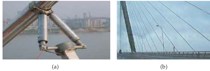
Figure 28: Dongting Lake Bridge with MR dampers.
