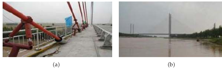
Figure 29: Binzhou Yellow River Highway Bridge with MR dampers.
