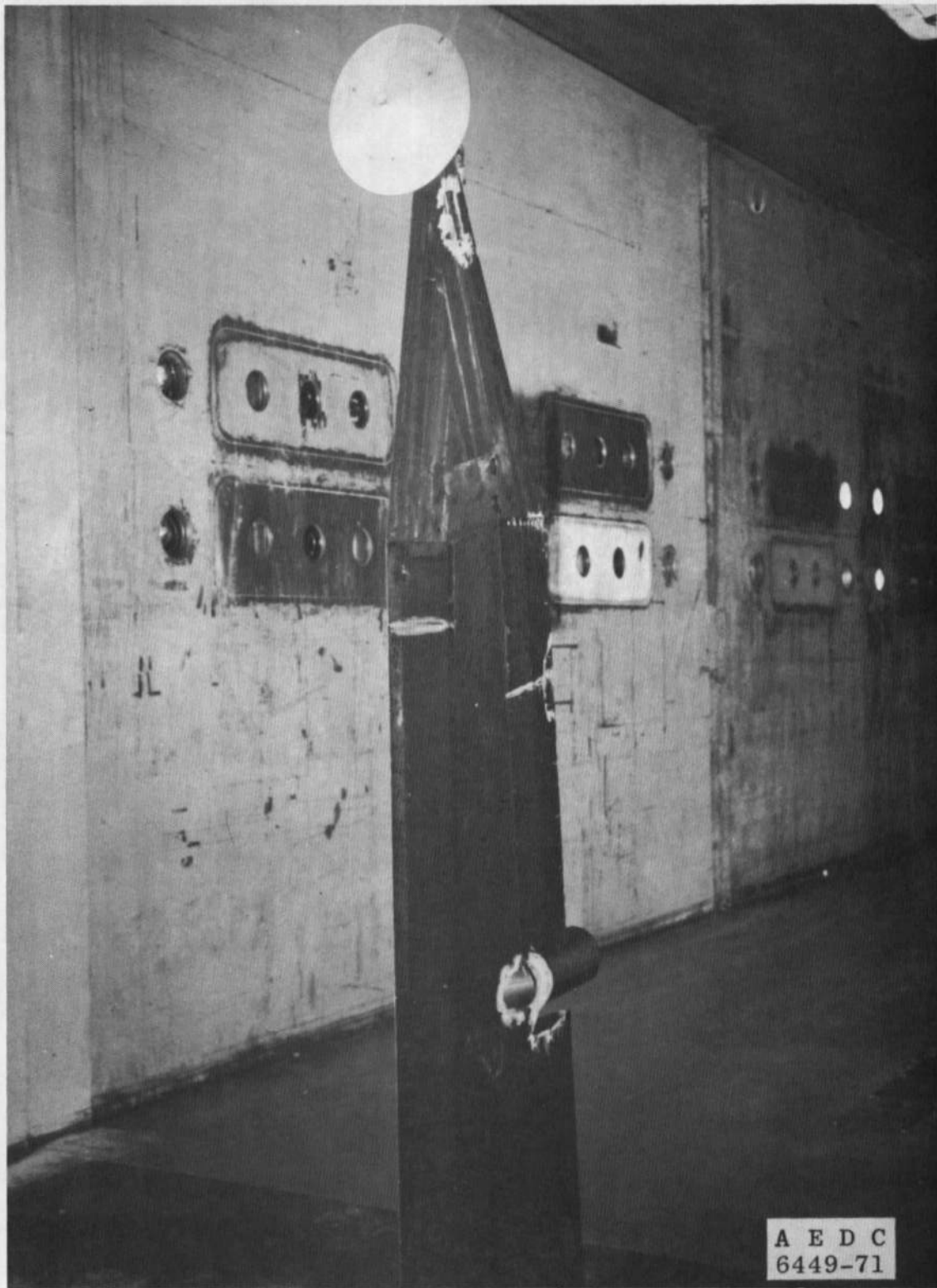
a. Entry Vehicle Model in Tunnel 16S Fig. 2 Installation Photographs
