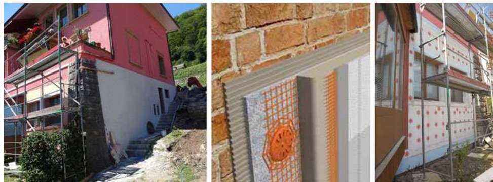
Fig. 25 Retrofit basement level insulation with Röfix AEROCALCE aerogel blanket insulation system. Building front/side-on view ( left ), cross section of the layered nature of the AEROCALCE system ( middle ) as well as ground level wall and window details ( right )
