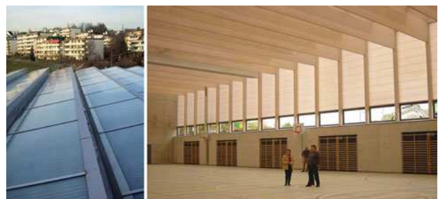
Fig. 19 First example of the use of Cabot aerogel granulate filled Scobatherm glass fiber composite panels in the form of a transparent daylighting roof construction is the gymnastics and physical education hall of the school Buchwiesen in Zurich which was constructed in 2003
