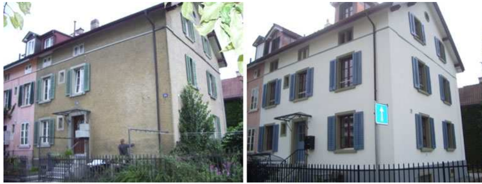
Fig. 23 Retrofit of an early 20th century city multifamily house in Zurich, Switzerland. Exterior appearance before ( left ) and after ( right ) the renovation
