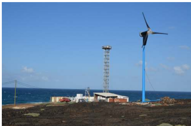
Fig. 1. CVAO station situated at the coastline of the Sao Vicente Island in the northern tropical Atlantic with clear view of the 30 m high measurement tower, some measurement containers, and a wind turbine for subsidizing electrical energy.
