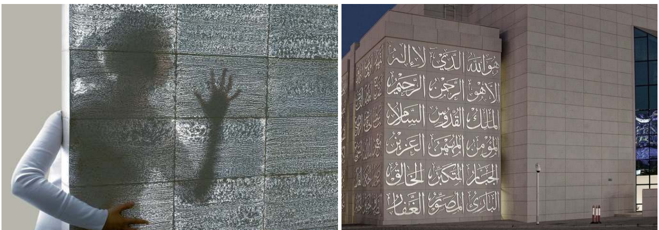
Figure 12. The previous practice of collaging glass and concrete materials next to each other is transgressed in the creation of light-transmitting concrete: left, precast building blocks by Litracon® (image source: Litracon®; reprinted with permission); right, Al-Aziz Mosque's light-transmitting façade (design, production, and photo by LUCEM Lichtbeton®; reprinted with permission).
