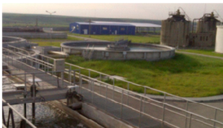
Figure 1. Alexandria wastewater treatment plant.
