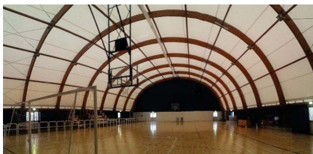
Figure 1: Air dome internal view
